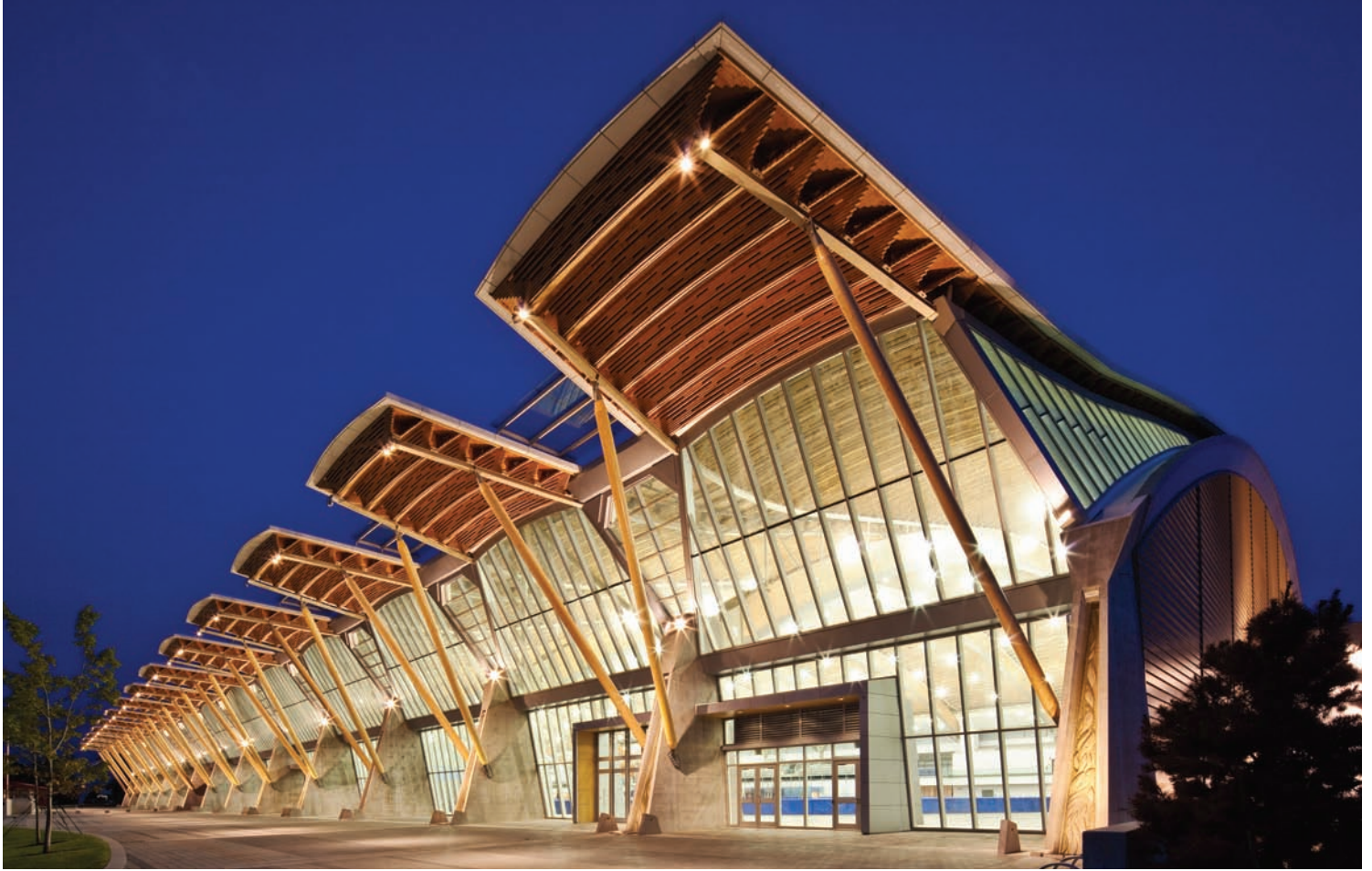
ABOVE A PHOTO OF THE FACILITY'S EXTERIOR ILLUSTRATES THE ENORMOUS CONCRETE BUTTRESSES REQUIRED TO BRACE THE 110-METRE-LONG GLULAM BEAMS.
